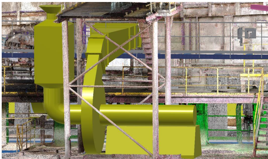
Figure 3. Example of collision check in laser scan point cloud.
